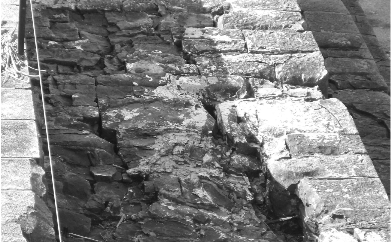
Gilboa Dam: Visible deterioration
