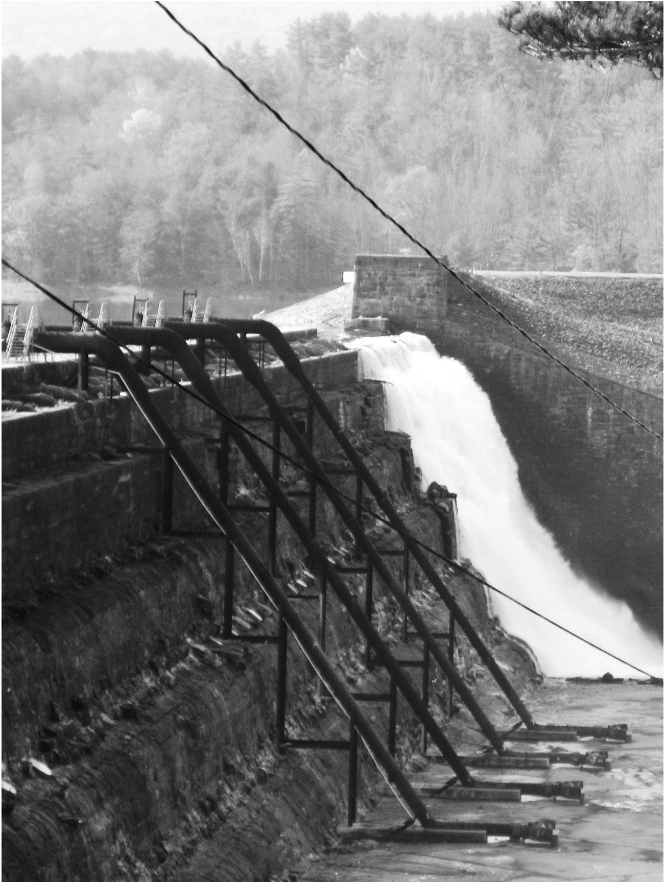
Gilboa Dam: Siphons and a notch cut into the spillway are features of ongoing interim repairs.
